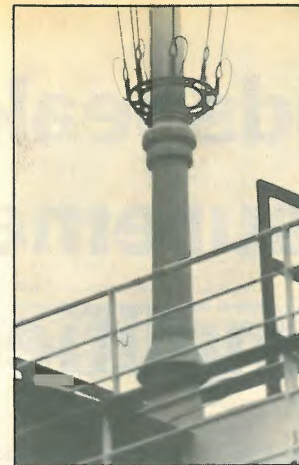
Fig. 11. Base of Russian mast showing three deep-skirted rain cones on the central glass-fibre pole. (Photographed at Rouen, 1983.)
